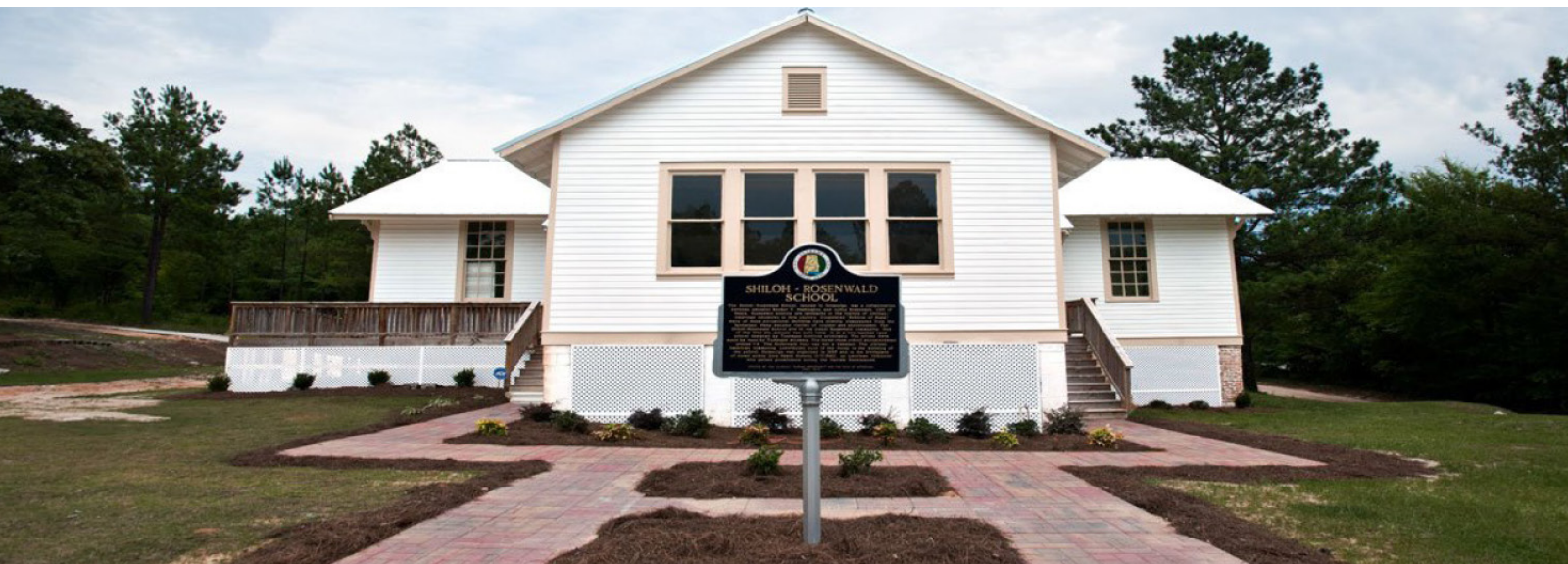
Above: Renovated Shiloh-Rosenwald School, Notasulga, Alabama. (Photo: Darrell Moye)
